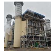
NPPMCL, HEI & GE announce completion of Balloki Power Plant
